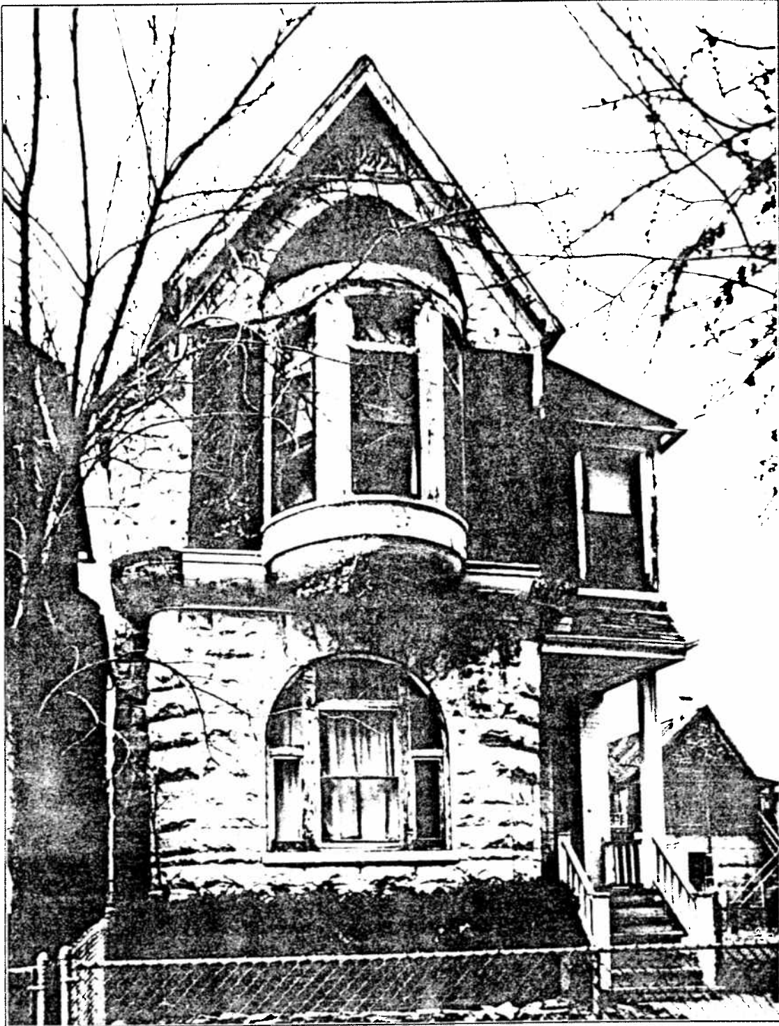
Figure 21: The house at 4160 South Lake Park Avenue. The design of this structure is typical of those by Hine on Lake Park and Berkeley. With its first floor of rusticated stone and with its second floor in frame "simple work," this house exemplifies the development as it was described in the Chicago Inter Ocean in January, 1887. (Photograph by Raymond T. Tatum)
